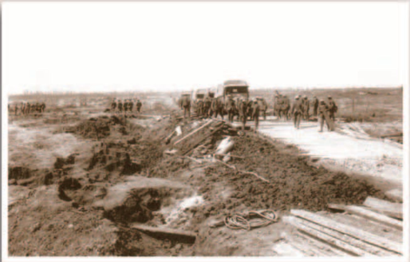
Building a plank road through the mud. [LAC PA 1226]
