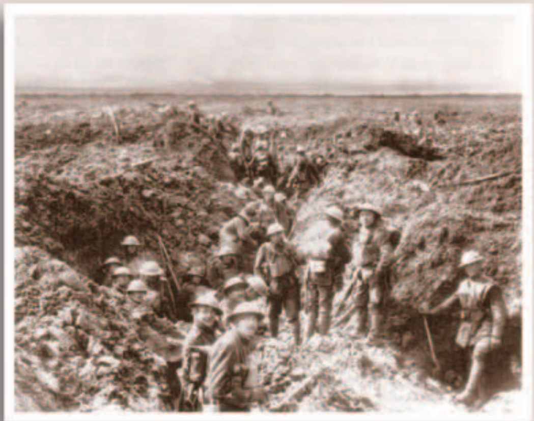
Holding newly-won ground was often more difficult than taking it. Canadians dig in just behind the eastern rim of the crest. [LAC PA 1085]
