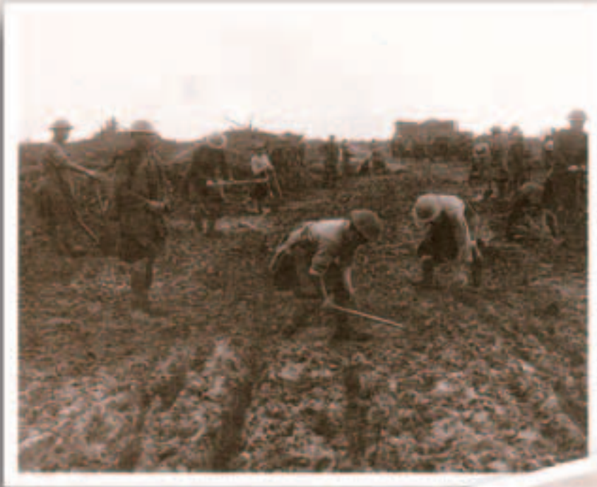
Canadian "highlanders" work with pick and shovel to build a road over shell-torn ground. [LAC PA 686]
